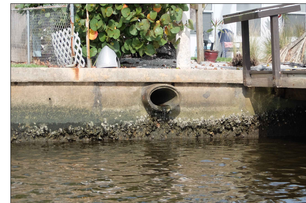
PHOTO OF EXISTING CONDITIONS N.T.S.
